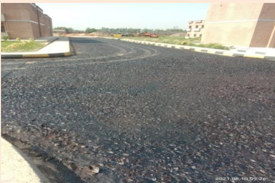
Prime Coat Completed
